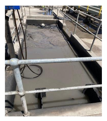
Photo 11 – Oily water separator located near the wheel washing station appeared to be approaching capacity
