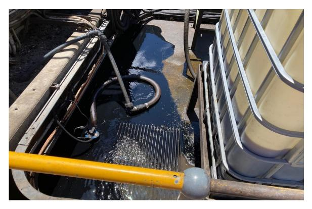
Photo 10 – Drain blockage located in the fuel farm bunded area filling with hydrocarbon contaminated water
