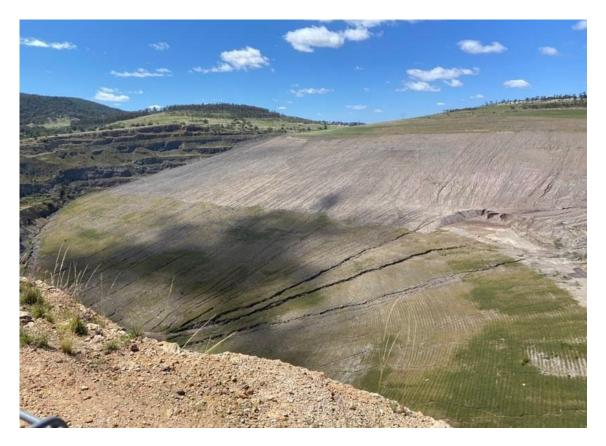
Photo 6 – Extensive rilling and scouring in areas of completed rehabilitation in Open Cut 2
