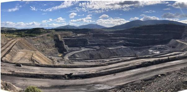
Figure 40: Photo of Open Cut 1 showing effective Spontaneous Combustion Management
